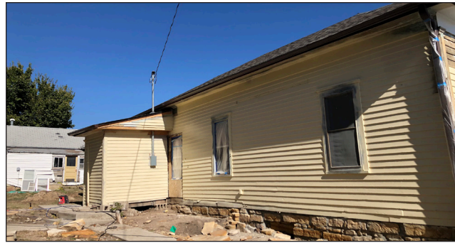
Back of house prior to foundation repair and dirt work
