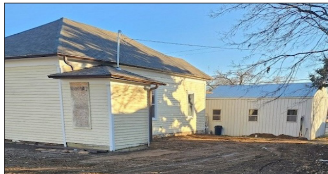
After dirt work completed
