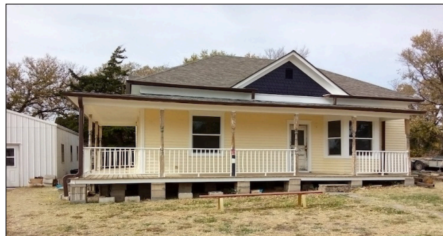
East side painted
